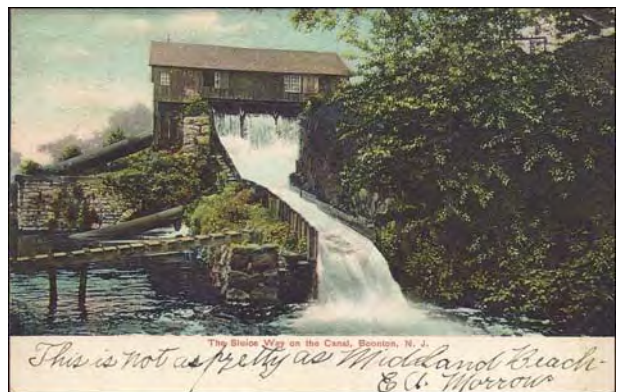
Fig. 20: The Sluice Way on the Canal, Boonton, N.J. Excess water being returned to the canal. (Machine cancel, Boonton NJ, October 30, 1907; received Paterson, NJ, October 30, 1907 machine cancel.)
