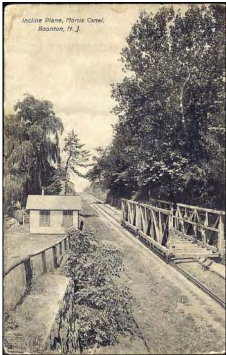
Fig. 21: Incline Plane 7E, Morris Canal, Boonton, N.J. (58.60 miles). The wooden structure on the rails is the carriage which held the canal boat as it moved on the plane. (Machine cancel, Boonton, December 13, 1907, receiver cancel Manasquan, NJ December 1907.)
