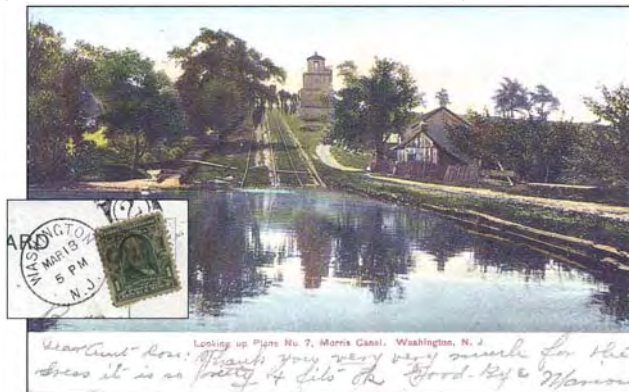
Fig. 14: Looking up Plane No. 7. Morris Canal, Washington, N.J. Plane 7W (14.75 miles) lifted the boat 73 feet. The cupola building is the power house holding the water-powered turbine used to pull the canal boat up/down the incline. The large basin at the bottom of the plane was used to hold boats waiting to go up the plane. (Hand cancel, 2nd class office, Washington, NJ, March 13, 1912.)
