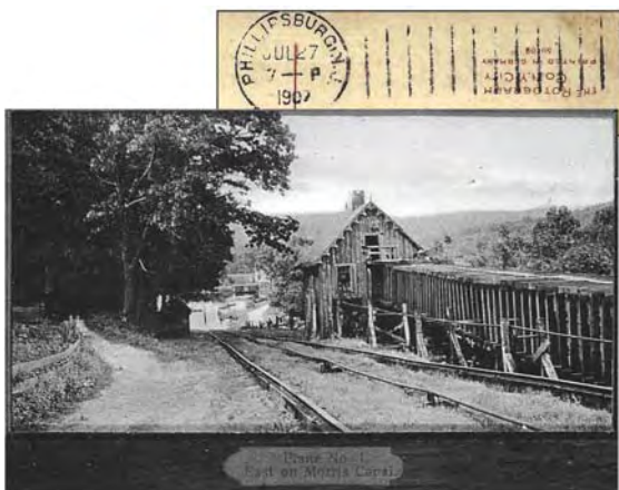
Fig. 19: Plane 1 East on Morris Canal (39.90 miles). Long wooden structure leading into the powerhouse carried the water to operate the turbine to move the boat up/down the plane. (Card cropped to show view.) (Indistinct postmark, Barr-Fyke received machine cancel Phillipsburg, July 27, 1907.)
