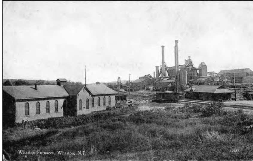
Fig. 30: Wharton Furnaces, Wharton NJ. Plane 5 East was adjacent to the Wharton Furnace (47.00 miles). (mint)
