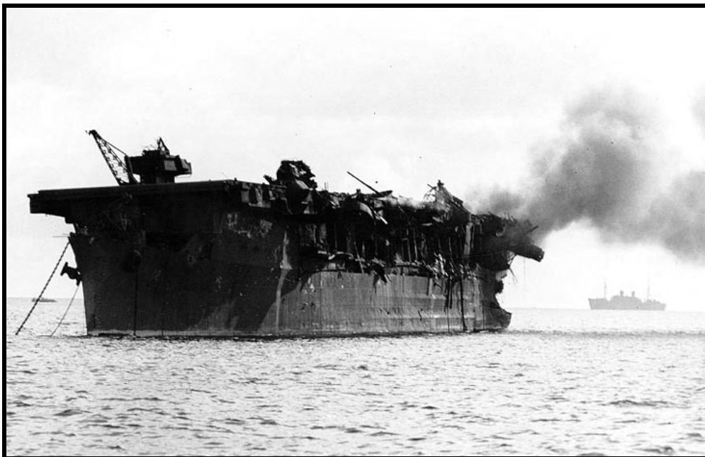
Fig. 25: USS Independence, afire aft, soon after the "Able Day" atomic bomb air burst test at Bikini on 1 July 1946. The bomb had exploded off the ship's port quarter, causing massive blast damage in that area, and progressively less further forward.
