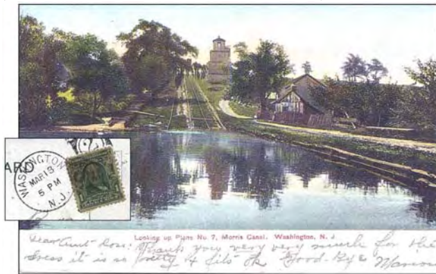
Fig. 14: Looking up Plane No. 7. Morris Canal, Washington, N.J. Plane 7W (14.75 miles) lifted the boat 73 feet. The cupola building is the power house holding the water-powered turbine used to pull the canal boat up/down the incline. The large basin at the bottom of the plane was used to hold boats waiting to go up the plane. (Hand cancel, 2nd class office, Washington, NJ, March 13, 1912.)
