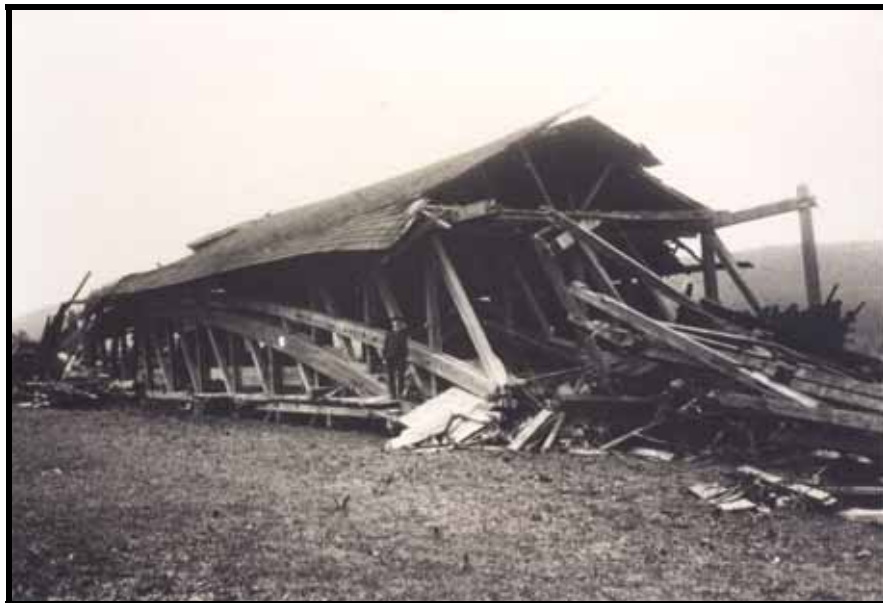
Fig. 2: Photograph of the remains of the old bridge following the flood on the Pennsylvania side of the river near Bowman's Hill, where it came to rest.
